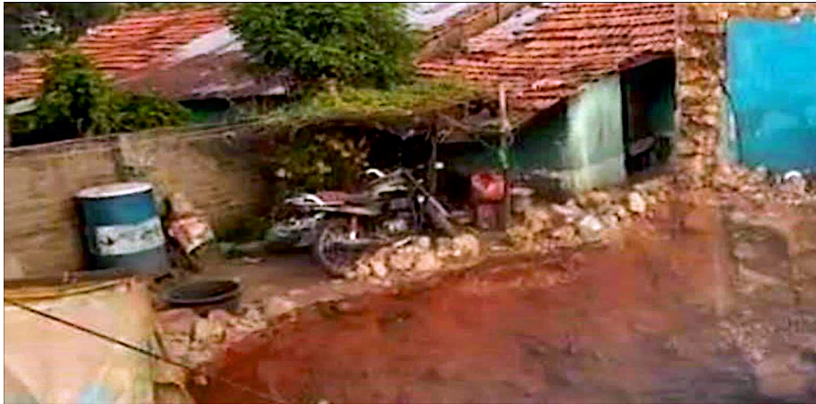
Figure 6: Sudden Collapse of a House in Ghugus City Due to Irregular Backfilling
